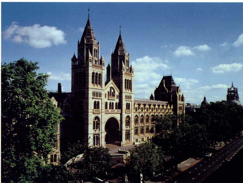
Fig. 1. The Natural History Museum, London, at the Cromwell Road entrance (view shows about half of front of building) (© 1999 Natural History Museum).
